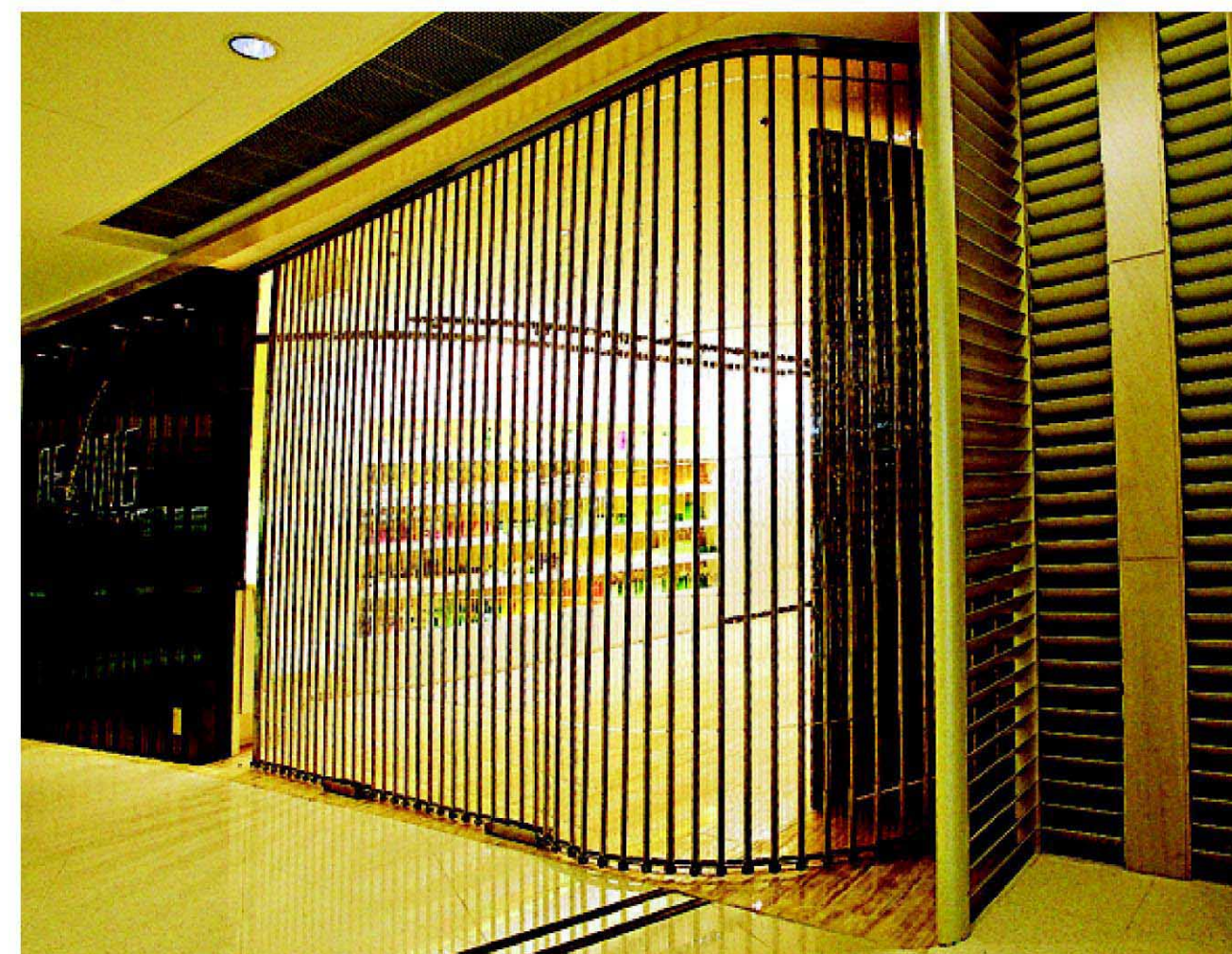
Clearseal IIs laterally sliding shutter in shopping arcade Elements, Kowloon Station
